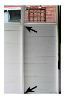
A good location will allow you to place the side brace close to a window or above the floor. The arrows indicate alternative positions for the side brace. We will use the top option in this shed. The Shackle itself will be between the arrows (see next photo)
